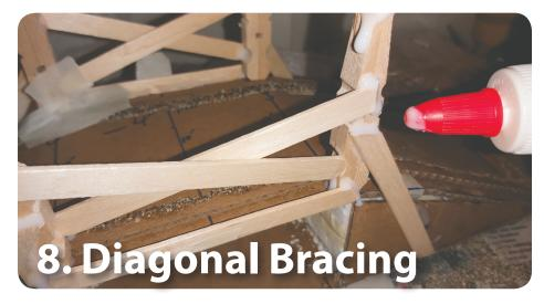
Use the details on the pillars to line up craft sticks. Test-fit, mark, cut and glue in place. Let dry. Add more glue on all the joints, flock with sand, and let dry again.
